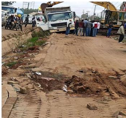
Figure 1: New road after 1 month.
