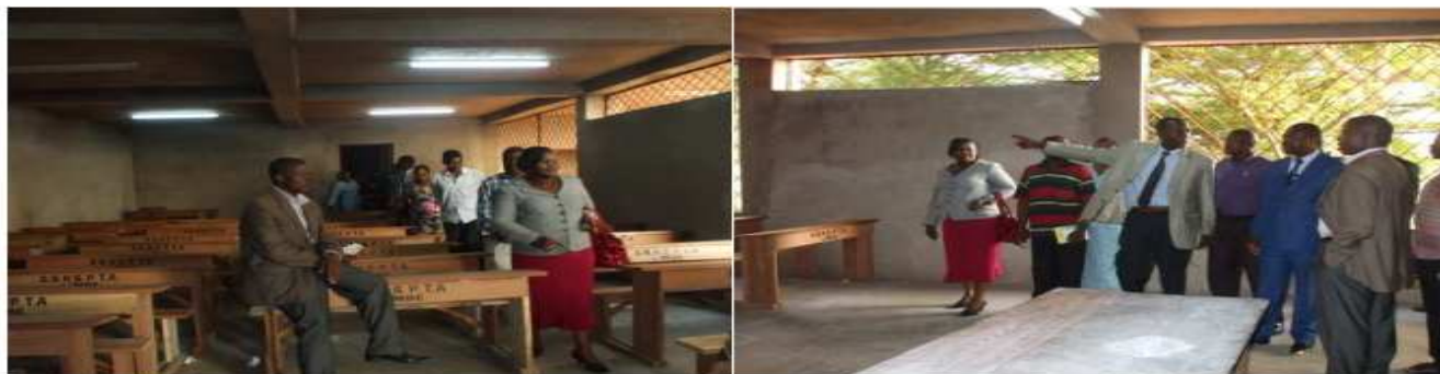
Control Team rates satisfactory the construction of classrooms financed through fees paid by Parents to GBHS Limbe
